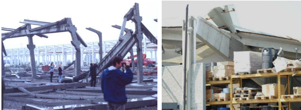
Figure 1: Damaged precast RC frames
