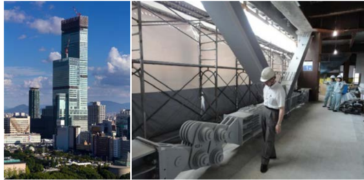
Figure 3. Japan tallest building with Rotation Friction Dampers
